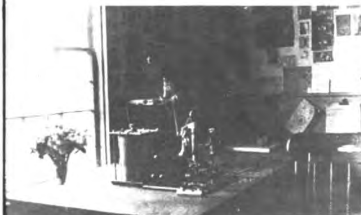
United Wireless Station "PM" at Eureka taken circa 1911-12 showing 2 KW Spark and Helix.
